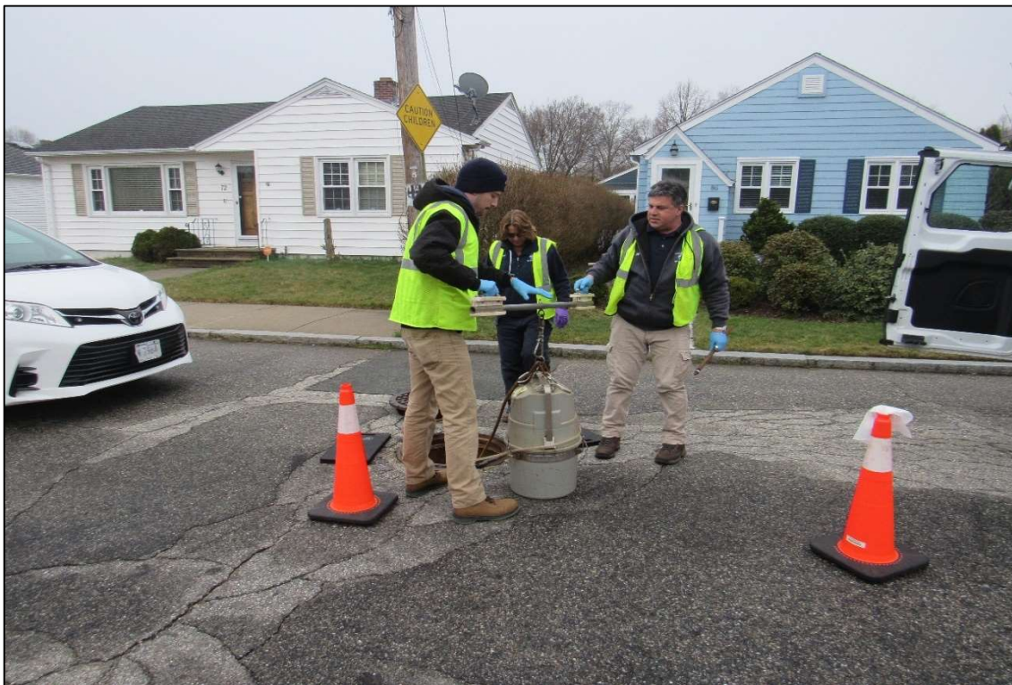
Environmental monitors conduct sanitary manhole sampling.
