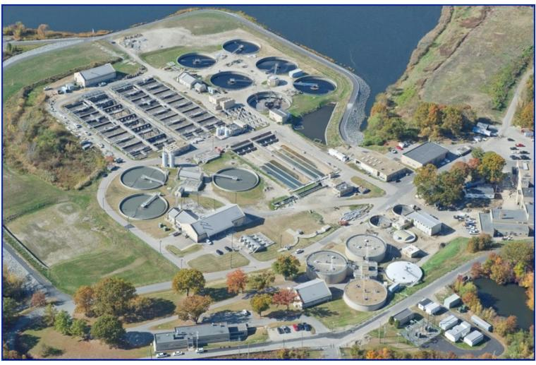
Field's Point is in Providence, RI. It has an advanced secondary treatment capacity dry weather) of 65 MGD. In 2021, influent flows averaged 44 MGD.
