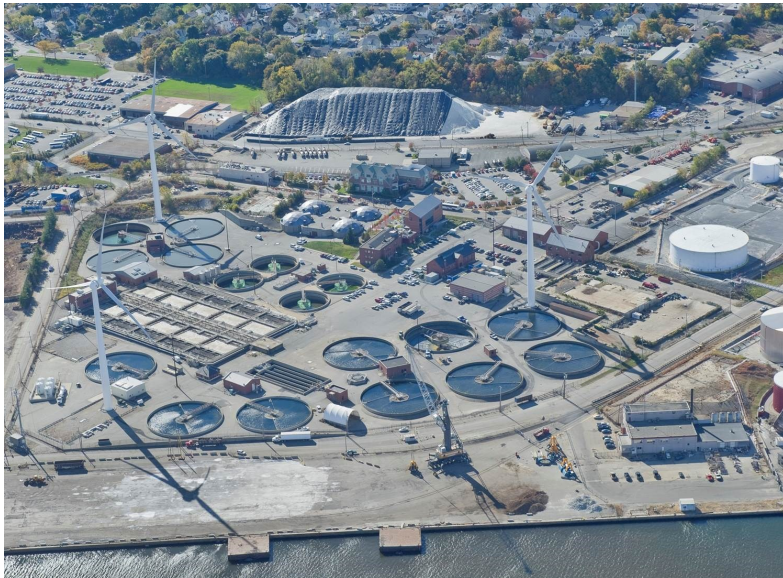
Aerial view of the Field's Point WWTF
